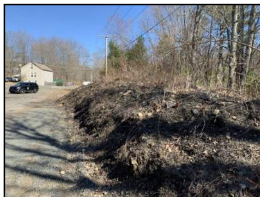
4 : A pile of fill material of unknown origin placed along the south side of the asphalt parking lot. View to the east.
