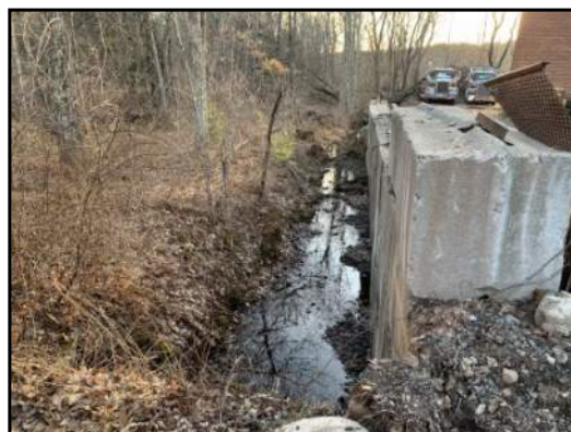
28 : Mill Race discharge to Furnace Brook. View to the southwest.
