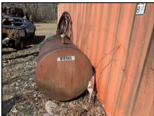
15 : Empty diesel AST (AST #1) along the west side of the shipping container. View to the north.
