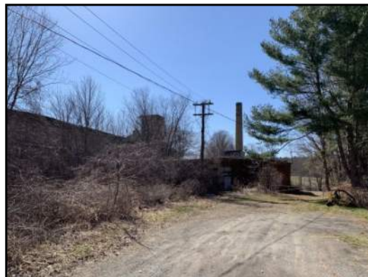
8 : Access along the north side of the Site. Pole-mounted power lines are not in service. View to the west, with the Mill Race along the left side of the photograph.
